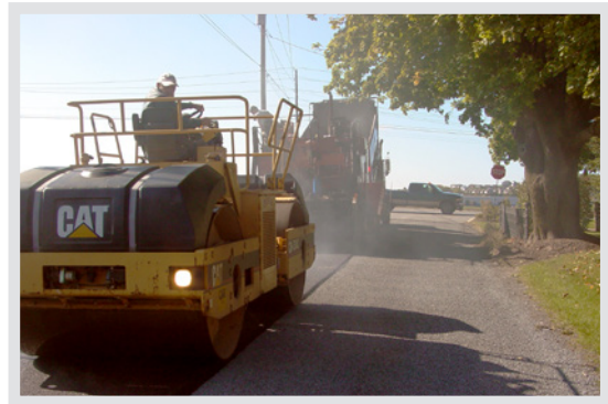
Second Step: Pave utilizing Open Graded Friction Course
