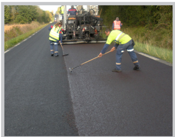
Nova-Surfacing application
