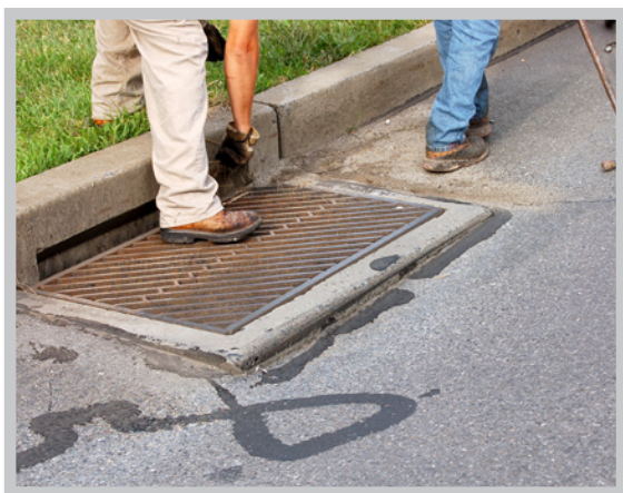
Cleaning surface in preparation of repair
