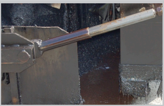
Polymer Modified Tack directly in front of Hot Mix
