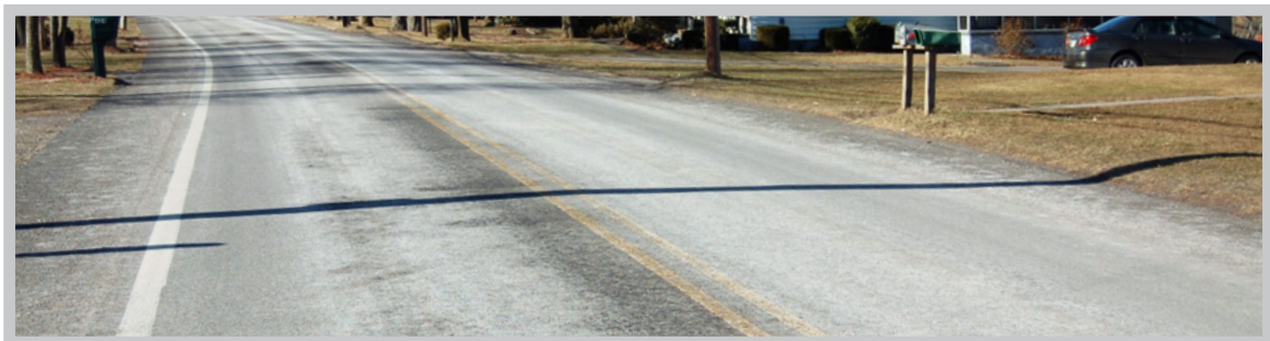
Open texture retains salt and may not require pre-treatment for next storm
