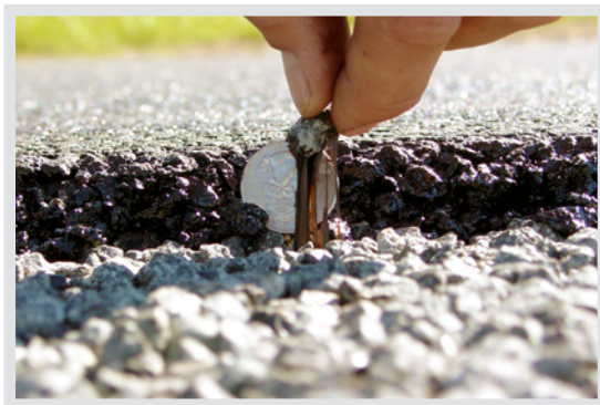
Note: 5/8" depth of paving & polymers in High Performance Chip Seal
