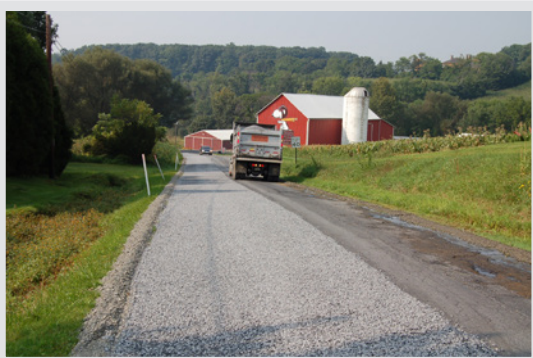
Course aggregate is Paver-Placed to correct profile
