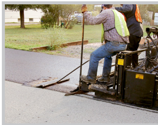
Slurry applied over High Performance Chip Seal
