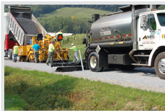
Emulsion applied at 1.5 gallons per SY
