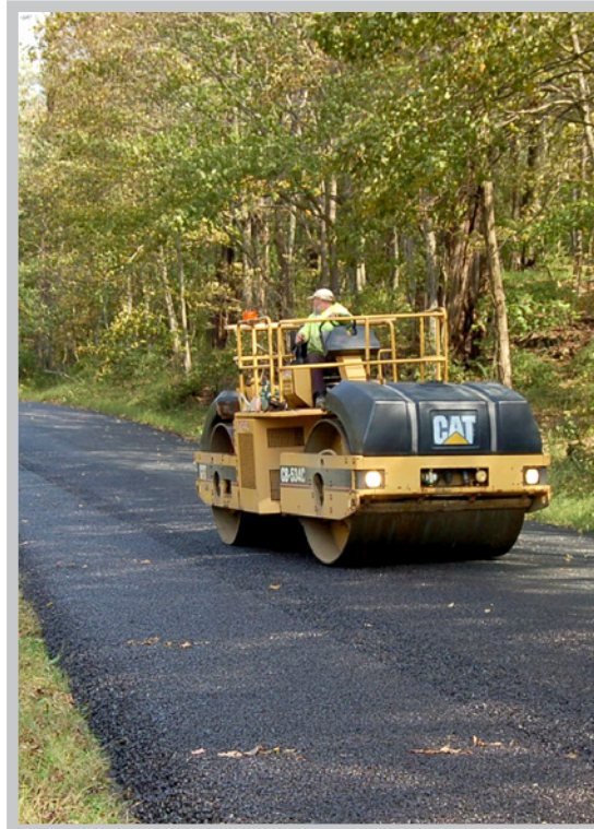
Compacted with 10 ton static roller
