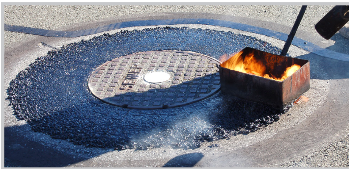
Flowing PolyPatch around manhole to make smooth transition from street to manhole
