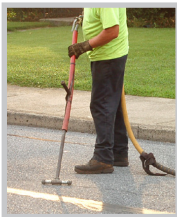
Close up of air cleaning cracks
