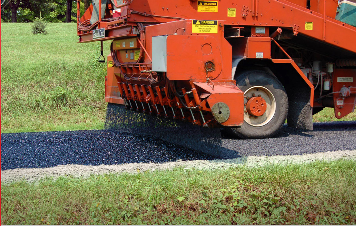
Fine aggregate spread across Paver-Placed course aggregate after application of asphalt binder.
