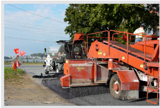
First Step: Place High Performance Chip Seal
