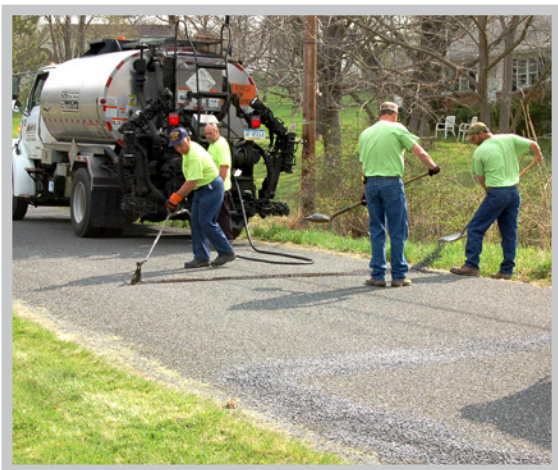
Asphalt Distributor - two people, rented equipment & labor
