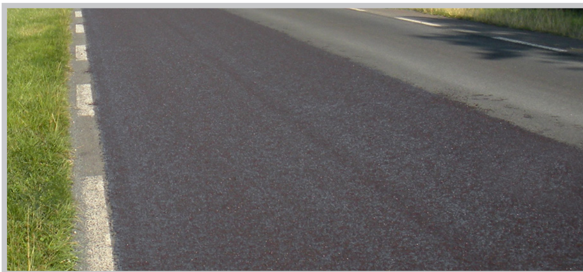
The macrotexture of the material creates a more flexible surface with improved skid resistance compared with Microsurfacing
