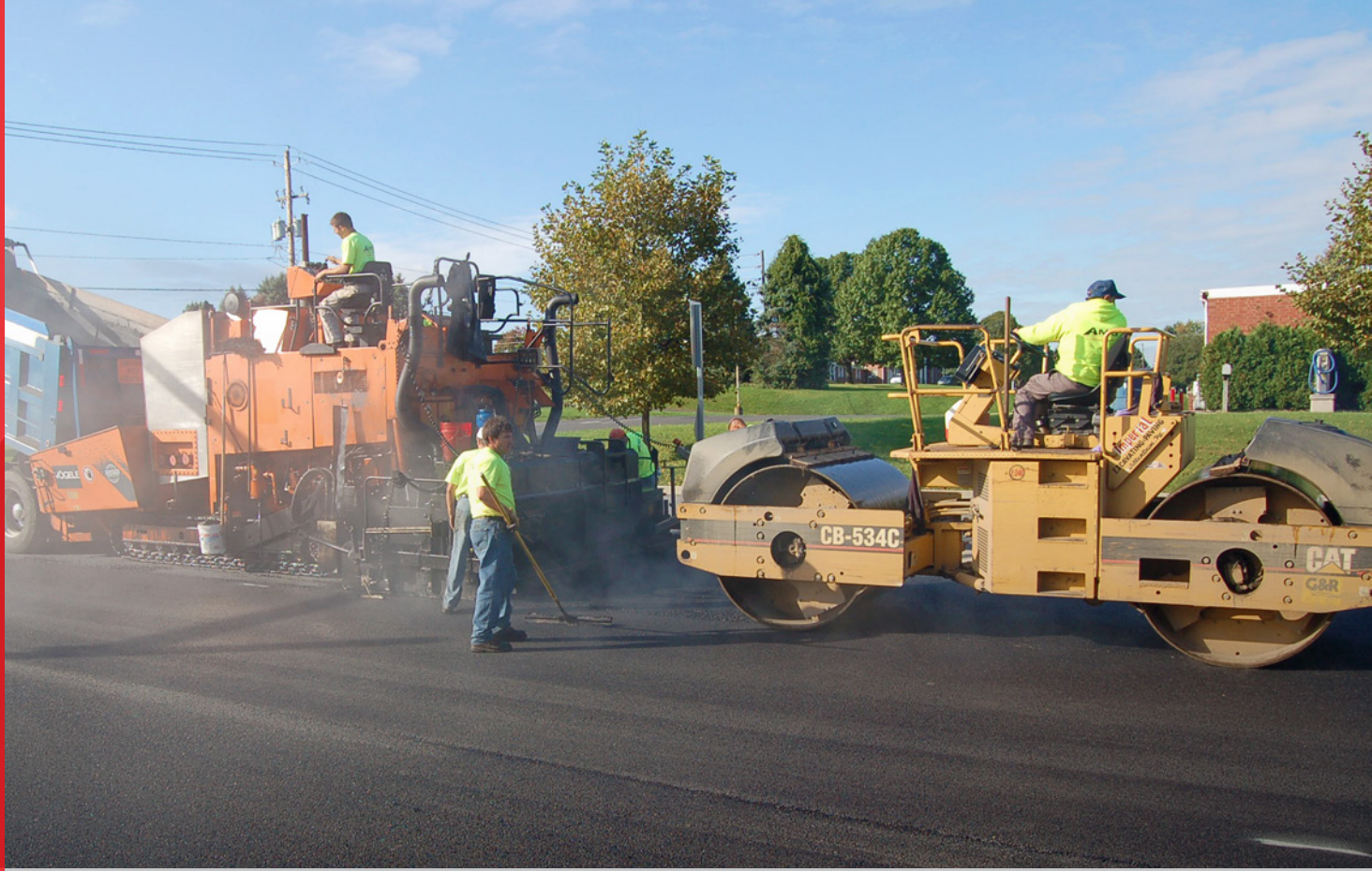
Special paver placing Ultra-Thin Friction Course followed immediately with steel finishing roller. Traffic can return as soon as the roller makes a single pass.
