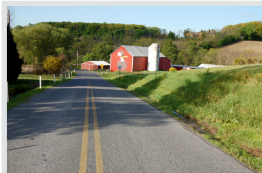
The same Double Chip Seal 5 years later
