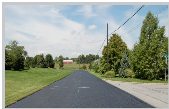
12 year old Ultra-Thin Friction Course after Fog Seal
