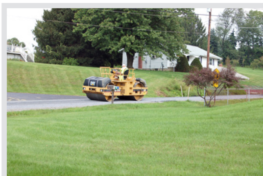
Rolled with 10 ton static roller
