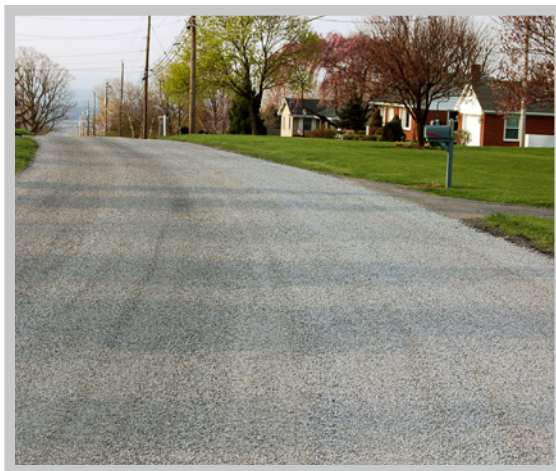
Road surface after Mechanized Skin Patching
