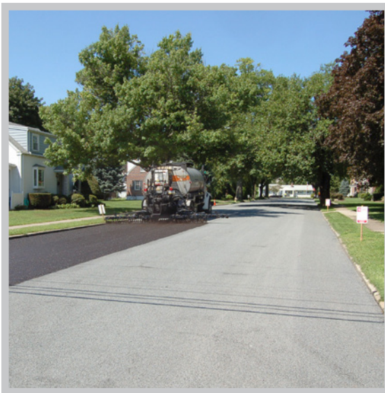
Grip Tight Fog Seal being applied to High Performance Chip Seal (City of Allentown)
