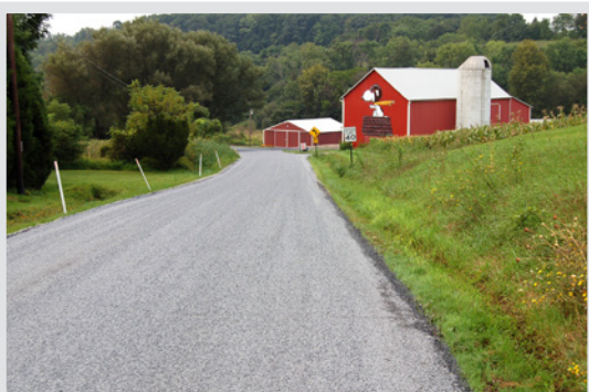
New finished surface with Double Chip Seal
