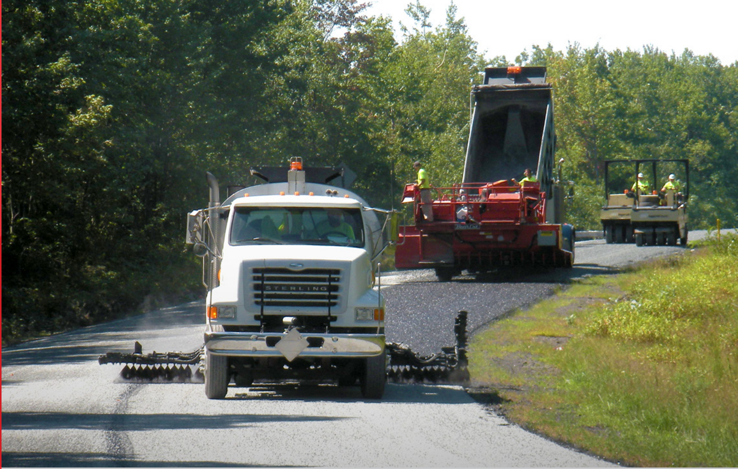
Second application of a Double Chip Seal (note tight pattern of equipment)
