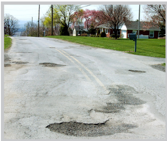
Road surface before Mechanized Skin Patching
