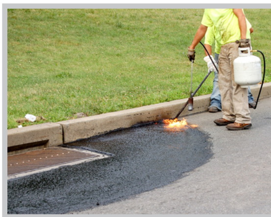
Completing patch by ironing joint
