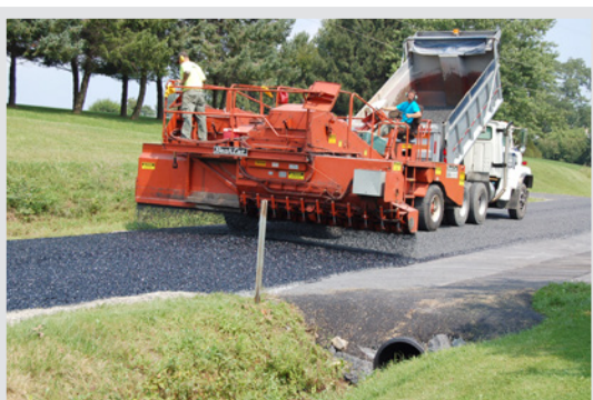
Fine aggregate placed with chip spreader
