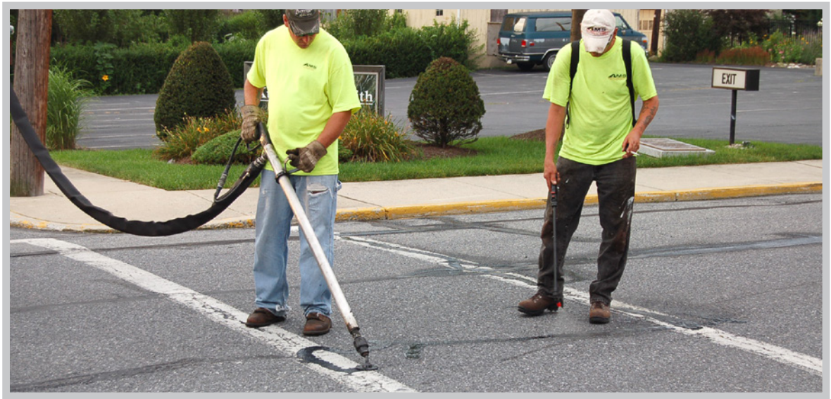
Applying Crack Sealer and immediately spraying De-Tack
